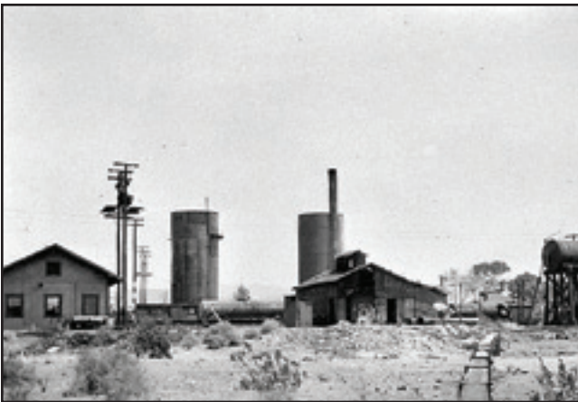
A 1923 photo of the Santa Fe railroad facilities at Bagdad.
